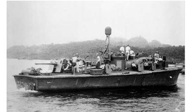
Browning Machine Guns (with steel armor shields) mounted near the chart house, and six (3 per side) single 50 cal. Browning Machine Guns (also with steel armor shields) mounted spaced along each side.
