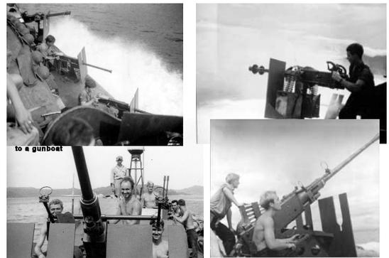
Both (existing) BMGs in the turrets also received steel armor shielding. Work on the 59 boat was completed on October 6, 1943 and moved to Rendova on October 8.
